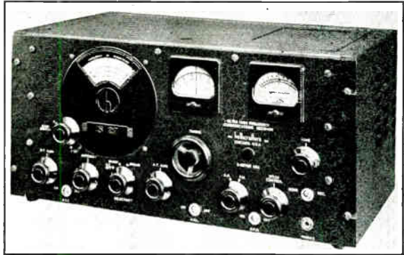
◆ Fig. 1120 — The Hallcraft S-27 u.h.f. receiver can be used for either a.m. or f.m. reception. The scale at the left indicates the frequency — the center scale is a vernier reading for accurate logging of signals. ◆
