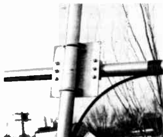
Fig. 14-55—The boom can be tied to the mast with muller clamps and a steel plate. The coaxial line from the driven element is taped to the boom and mast.
