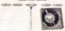
The doublet type of aerial is excellent for reception on short waves. The electrical interference and other noise picked up on the twin feeder is balanced out with a consequent reduction in background noise.
