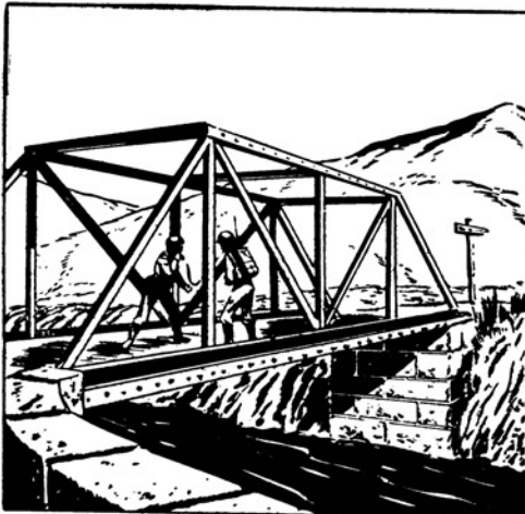
OVERHEAD STEEL BRIDGES
