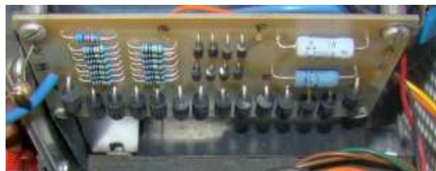
Figure 1.4 RM-220 Rectifier and Metering Board Upgrade
