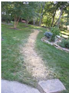
Trench Filled and new grass seeded
