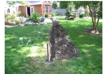
Trench for Coax
