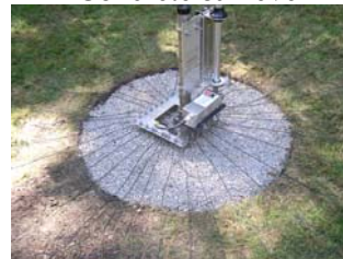
Radial Wires Installed Antenna Installed
