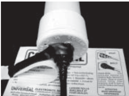
Apply one overlapping layer of Coax Seal. Press so that it sticks to the device and covers at least 1" of cable. The seal must be solid from device to cable.
