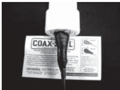
IMPORTANT - Make sure the Coax Seal is well whetted (stuck) to the device as well as to the cable.
