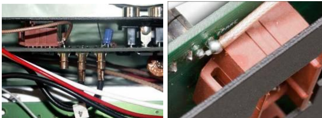
Figure 10: Spare jack connection (Photo at Right Courtesy of Roberto Barrios, EB4EQA)
