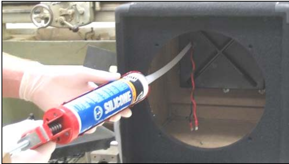
Apply RTV thru speaker hole in baffle
