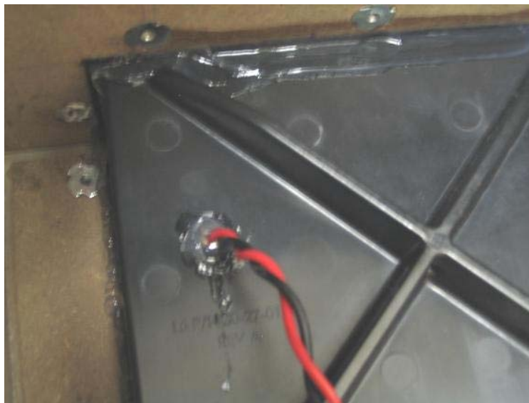
Finished RTV Application
