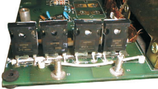
Figure 2.12. These four diodes need to be replaced.
