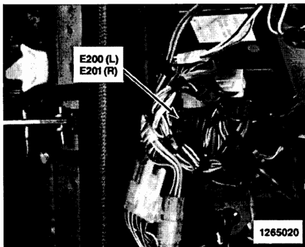
53. LH side behind footwell trim panel
