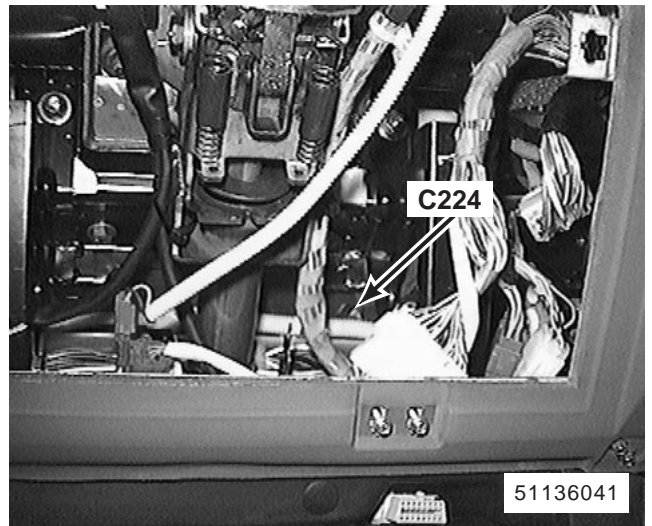
148. behind LH side of fascia right of steering column C224 (6-W)
