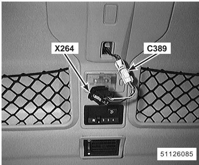
233. centre of roof X264 Passenger's Rear Sunroof Switch C389 (3-W)
