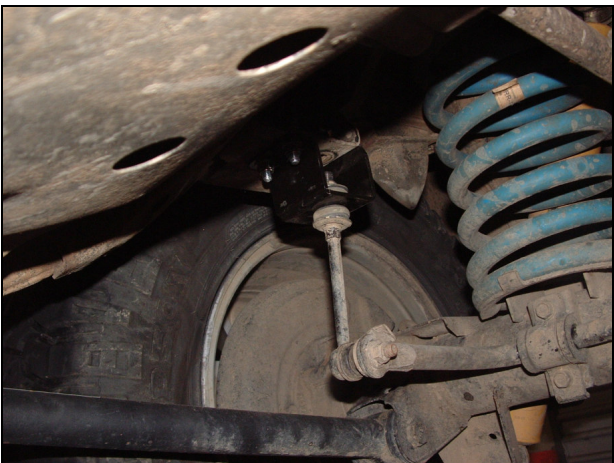
Right hand bracket installed
