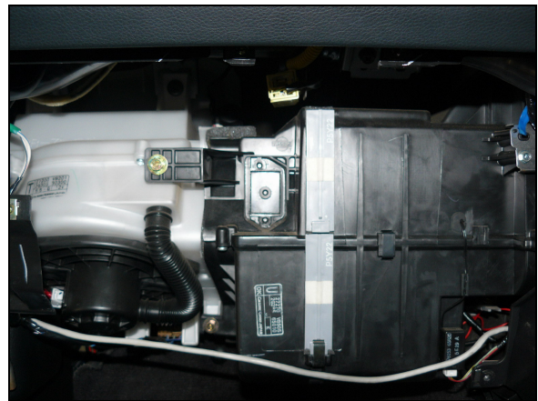
After the filters are installed
