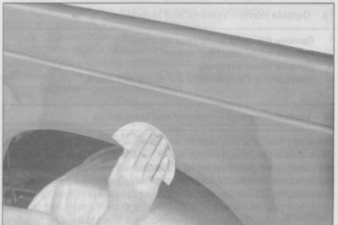
12 Finish sand the primer with very fine sandpaper (400 or 600-grit) to remove the primer overspray. Clean the area with water and allow it to dry. Use a tack rag to remove any dust, then apply the finish coat. Don't attempt to rub out or wax the repair area until the paint has dried completely (at least two weeks)
