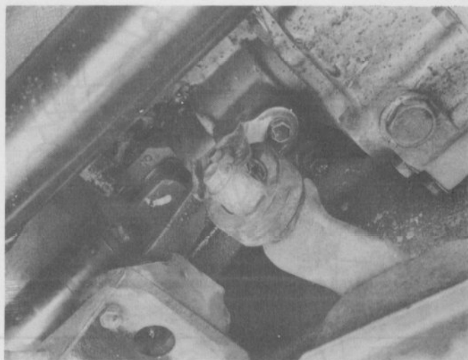
19.1c Here's a typical exhaust system hanger—these should be inspected for cracks and replaced if any are found
