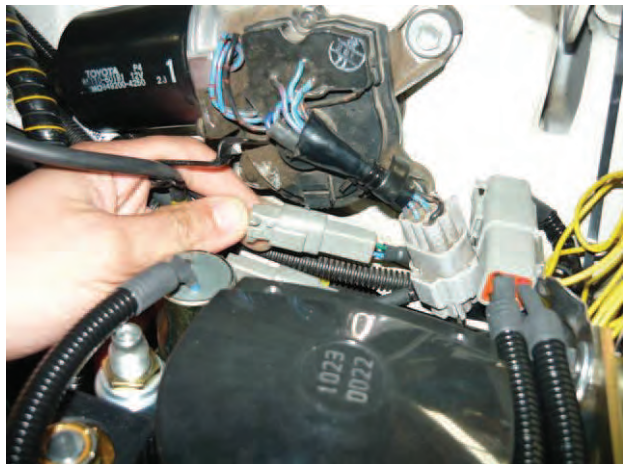
Figure 88: Connect the Power Box harness into the Cabin Control harness.
