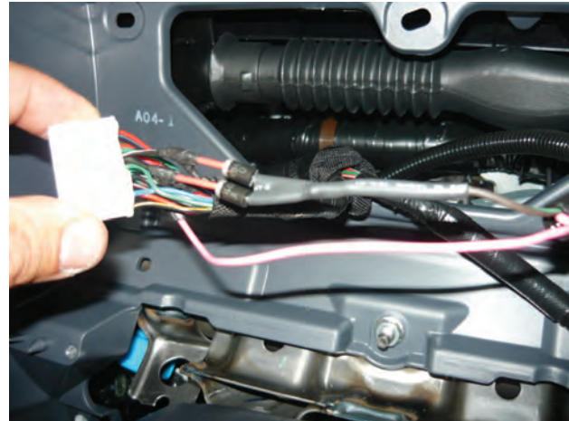
Figure 86: Insulate the joints with self-amalgamating insulation tape.
