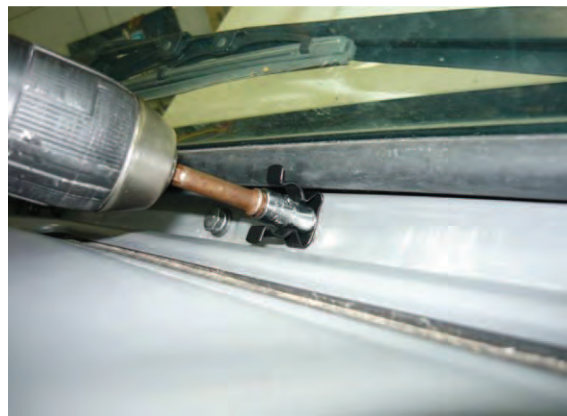
Figure 71: Fit clips using self drilling screws
