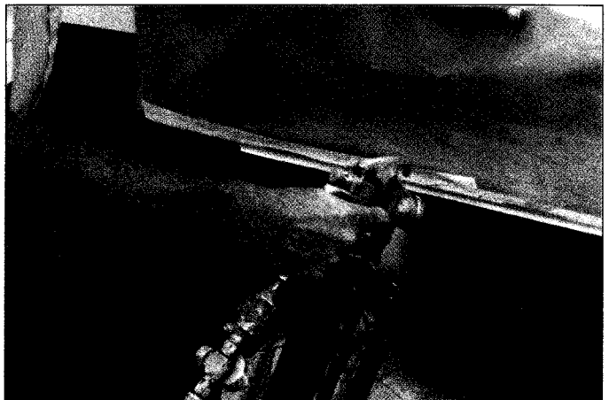
10 Apply several layers of primer to the area. Don't spray the primer on too heavy, so it sags or runs, and make sure each coat is dry before you spray on the next one. A professional-type spray gun is being used here, but aerosol spray primer is available inexpensively from auto parts stores
