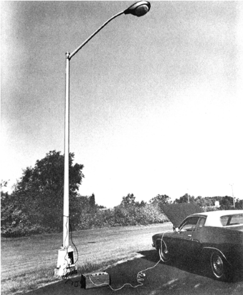
Figure 8: Testing Parking Lot Lighting; the Test Set Shown is Operating from an Inverter
