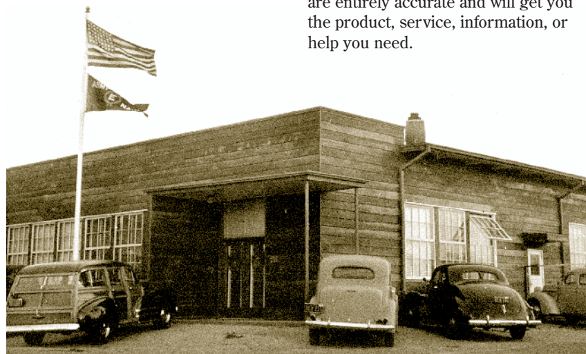
"The Redwood Building" at 395 Page Mill Road, Palo Alto, California. Hewlett-Packard's first company owned factory built in 1942.
