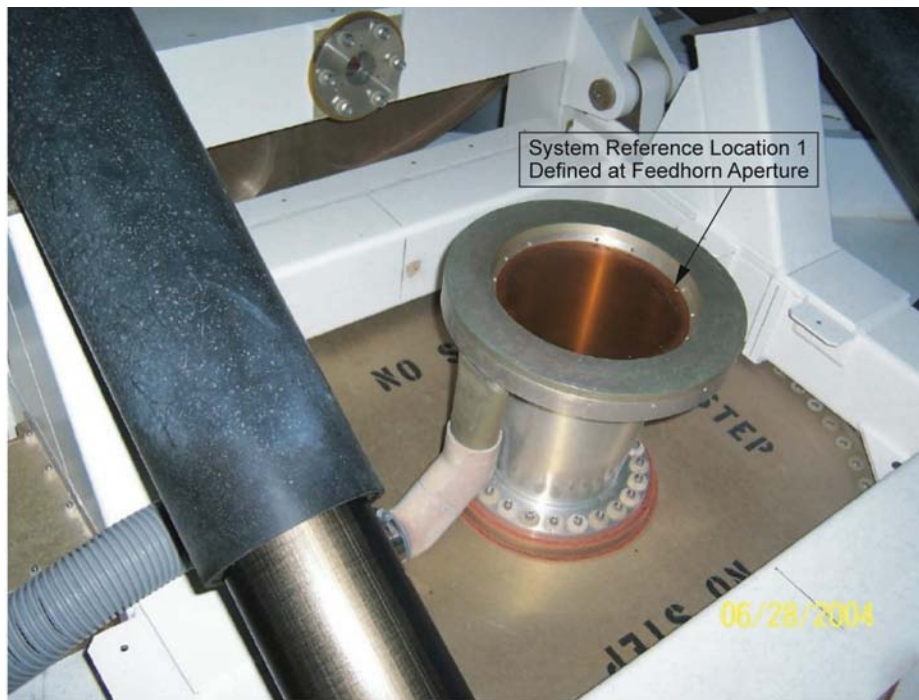
Fig. 2-8. Goldstone 70-m antenna XTR cone X-band feedhorn aperture reference location 1.
